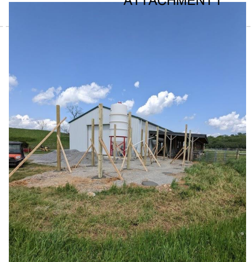
Southwest AREC Ram Barn Shed Extension in progress
