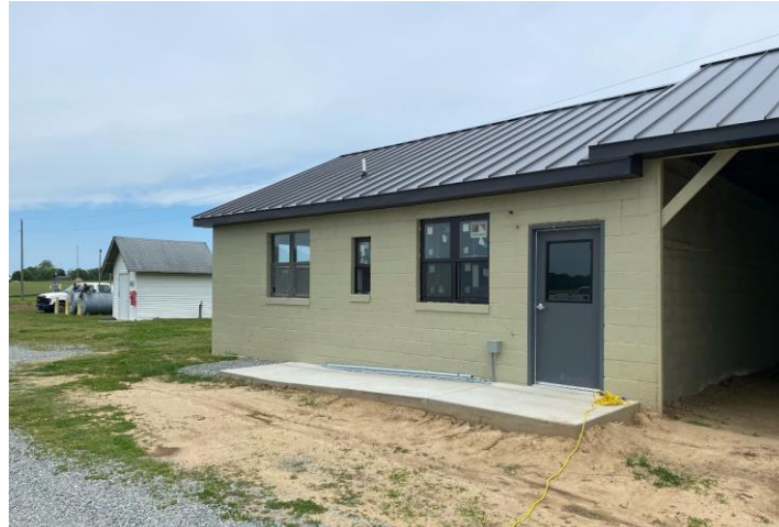
Eastern Virginia AREC Experiment Building Repairs
