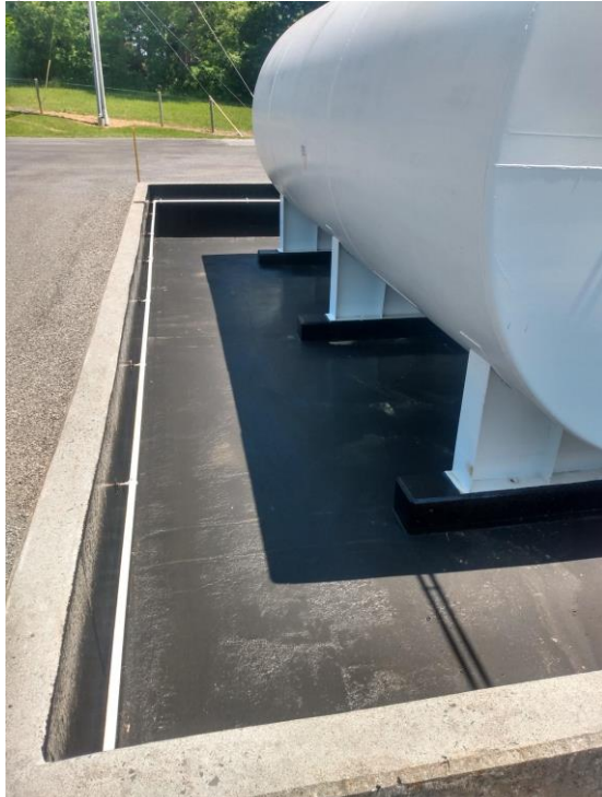
AHS Jr. AREC Fuel Containment Pit Repairs and Sealing
